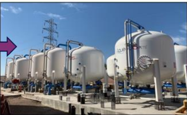
Granular Activated carbon (GAC) removes PFAS and any remaining hydrogen peroxide.
