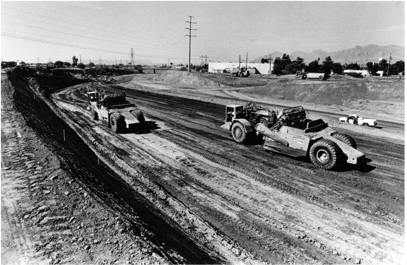
Road graders scrape the Santa Cruz River channel between Speedway and Grant roads during bank stabilization construction in May, 1991.
