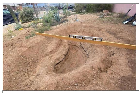
Gentle slope to the NW corner. Shelfs cut into the dirt to layer rocks on.
