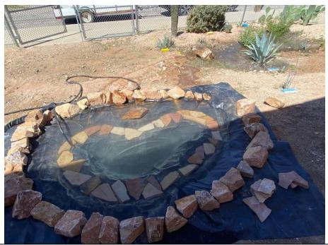
Fill the pond to check the fill height. Remove rocks and liner and repack the dirt to correct high or low spots. Make an intentional low point where you want excess water to go. Surround the pond with rocks of various sizes. Position rocks on pond ledges. Run the hose to overflow the pond and check for any low spots/leaks. Notice the overflow route.
